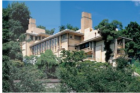
The Tazaemon Yamamura House near Kobe, built as a summer place for sake brewer Tazaemon Yamamura YODOKO STEEL WORKS
